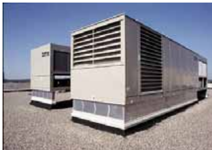
Applied Rooftop System
