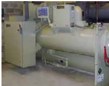
Single Compressor Centrifugal Chiller
