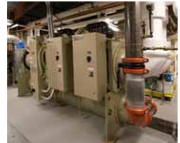
Magnetic Bearing Compressor Centrifugal Chiller
